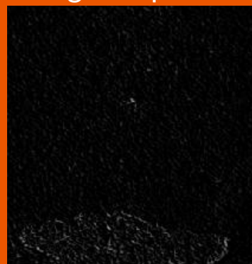
All edges of potholes
